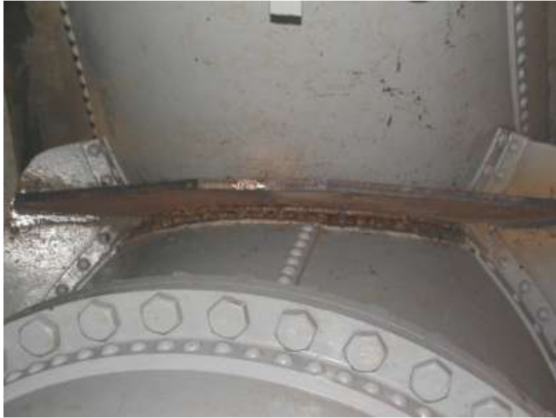
Strengthening fin at pipeline branching
