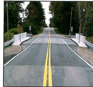
Photo 1: Geothermal Snow-Melt Bridge
