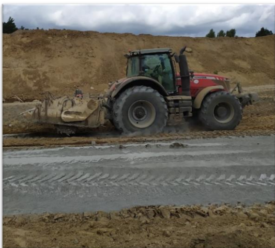
Fig. 3. Mixing the applied novel stabilizers with soil using conventional technique.
